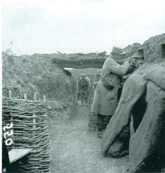
A glass view by LSU, No. 550 "Tranchee de 1re ligne" (A Trench of the front line). Taken in the early part of 1915, after the Horizon blue uniform replaced the dark blue overcoat and bright red trousers and field cap, and before the steel helmet was issued. One soldier stands guard with his rifle in a loop hole that is made of wood and built into the parapet of the trench. The soldier to the rear is stooping under a bombproof shelter. This was mainly a shelter from the rain
