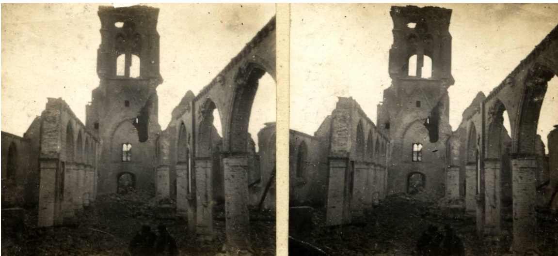
15. Pervyse Church Tower.
