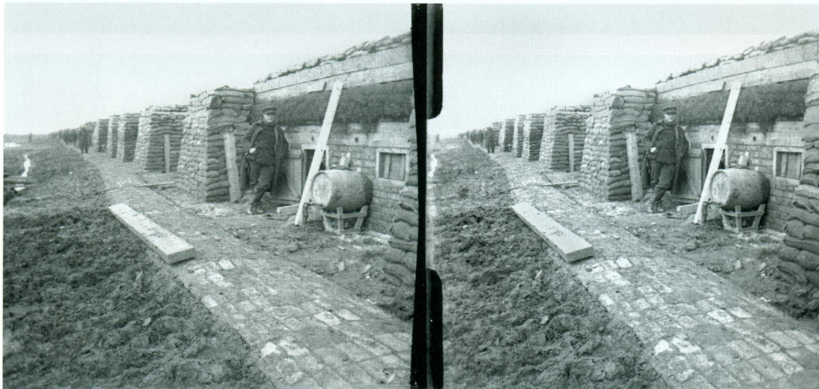
An above ground trench in Belgium. This is probably a 2nd or 3rd line trench, in a photo taken in 1915. The water table was so close to the surface that trenches in parts of Belgium could not be built in the ground, but were built above ground. The idea seems insane even for WW1, but they were not uncommon when water was close to the surface. Enemy artillery fire constantly tore them to pieces, and they were constantly rebuilt. It was a common practice if one's trench was even
