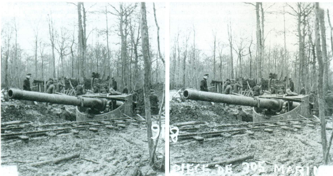
"Pierce de 305 marine" (305mm Naval Gun). A French glass view by an unknown maker of a 305mm, 12", naval gun with a naval crew. The gun is set on a rotating mount as if on a ship, and is anchored to a concrete base. There is a light gage railway line next to the gun to bring up shells and the propellant charge for the gun. It was not uncommon for navy personnel in the French and German fleets to be transferred to duties in the field after 1916, when the casualty rates were higher than the number of replacements available. The navy was the senior service in England, and very few navy personnel were transferred to duties with the army.
